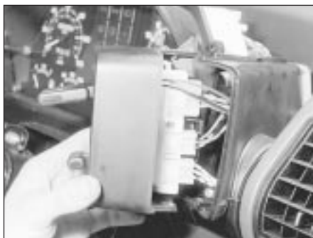
13.5A Withdrawing switch panel
