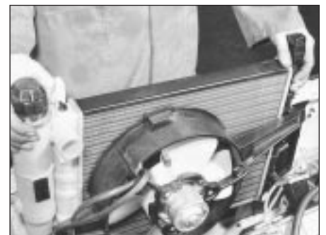
7.4B Removing radiator/fan assembly
