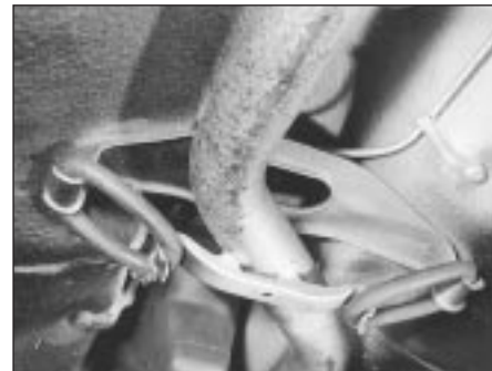
19.7A Exhaust pipe support rings
